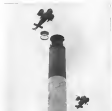
LIFTING THE LANTERN —An HO4S-1 (Sikorsky S-56) from the Second Marine Aircraft Wing places a 1100-pound lantern atop a new 140-foot lighthouse at Cape Fear, N. C., with only 8 inches of clearance on the sides. Hovering stability for this difficult job was provided by Sikorsky's Automatic Stabilization Equipment in the HO4S-1.
